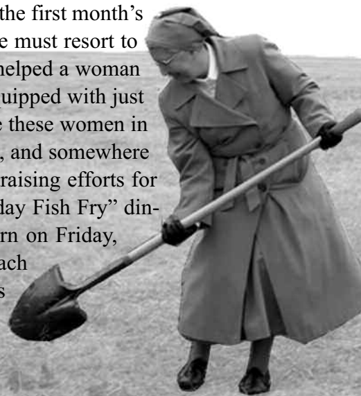
Sr. Jacqueline Darner helps break ground for St. Gianna Women's Homes facility
